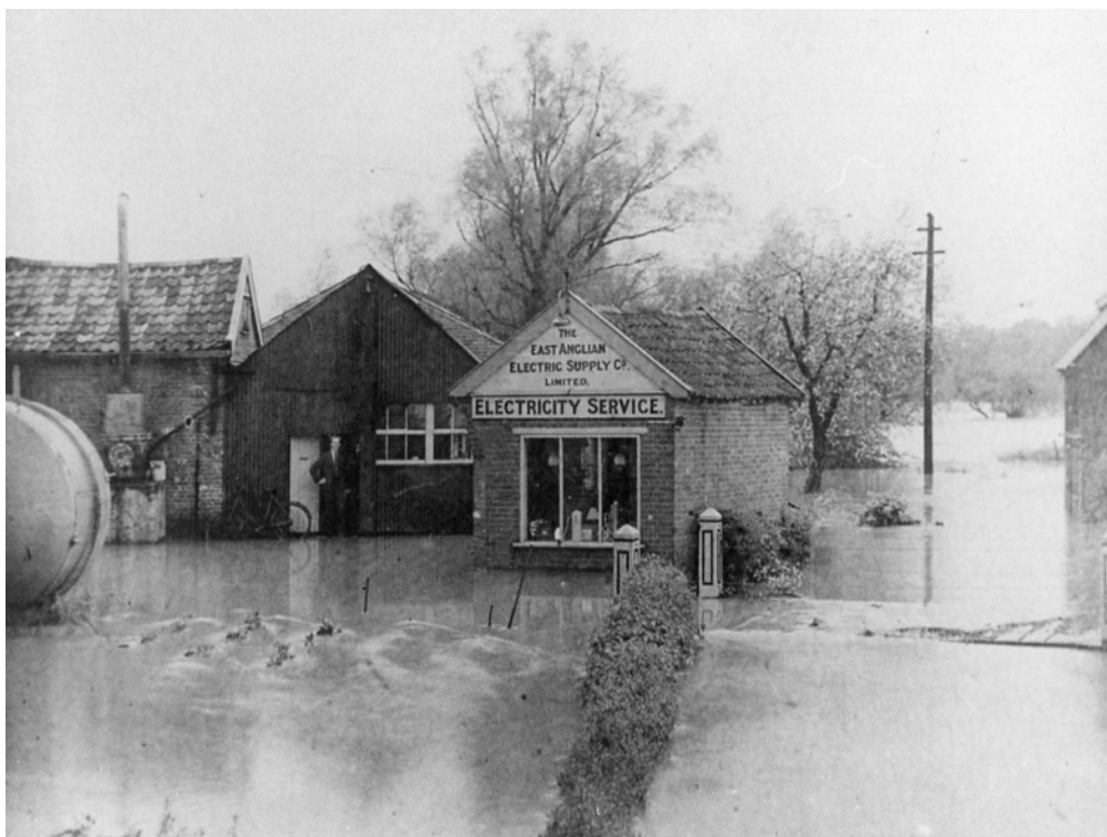
The Framlingham generating plant was in the old tan-yard buildings, and subject to flooding, 1938 Author's collection
