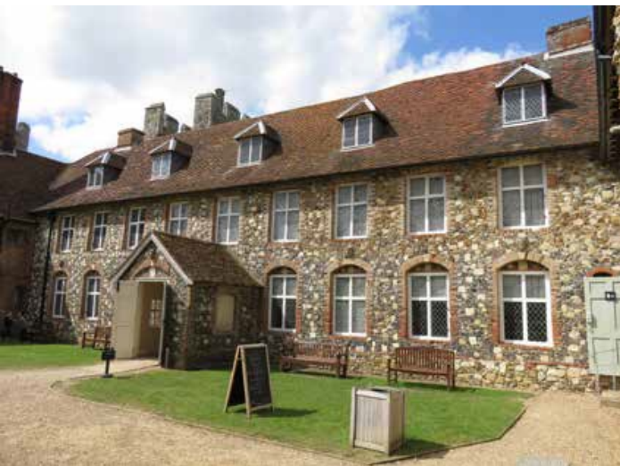
Fig. 6 The 1729 workhouse block, from the north-east. (© Historic England, K. Morrison)
