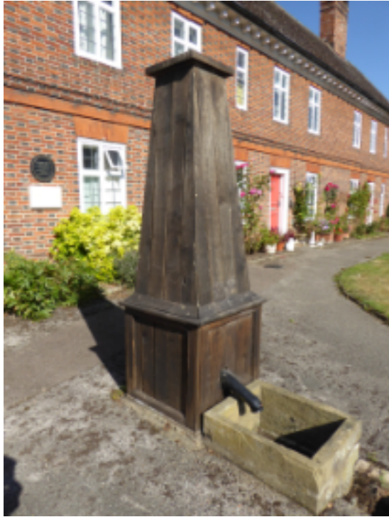
The enclosed pump, Mills Almshouses, 2020.
