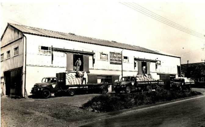
Clarke's cuber plant in Station Road
