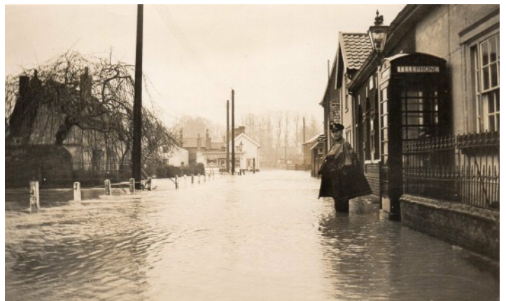
Floods in Riverside 1937. The gas lamp, telephone box and railings are all long gone.
