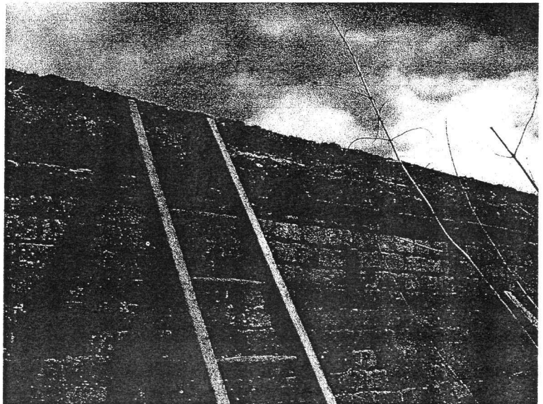
Figure 15. West wall of Langham Hall walled kitchen garden, showing slate drip line
